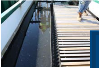
An operator can walk on the Drop-In to inspect, wash or replace the individually removable plates while the system continues to operate.
